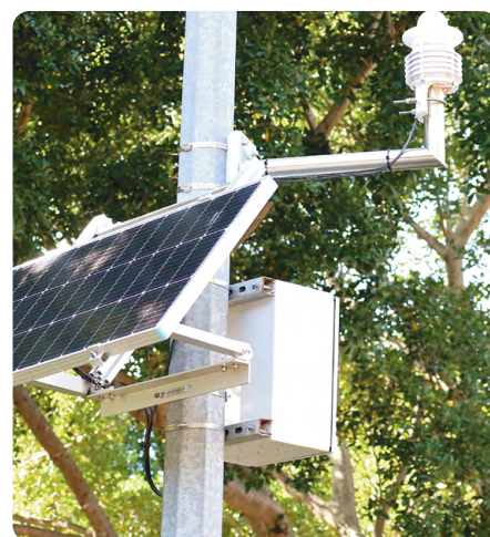
Environmental data is collected using weather stations installed throughout the park, to inform the SIMPaCT models that generate irrigation commands.
