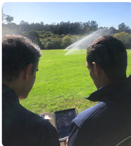
Irrigation controls and the SIMPaCT dashboard are accessed remotely via apps and websites.
